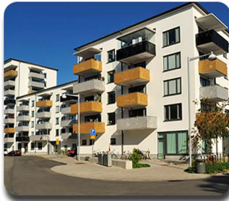
Civil building insulation
